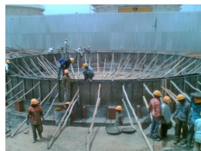
Installation of MMO ribbon
